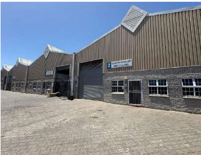
Photo 1: External view of Unit 2 in the Marconi Estate, leased by SGR
