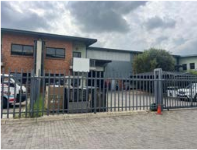
Photo 1: External View of Unit 17
