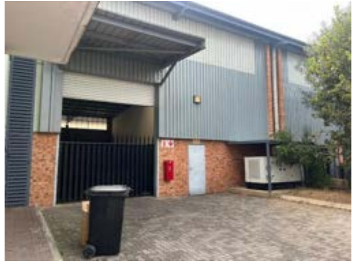
Photo 2: Unit 17 External View of Unit 17
