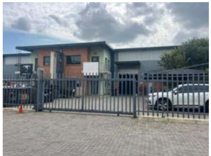
Photo 2: Entrance to Unit 17 of the Linbro Business Park
