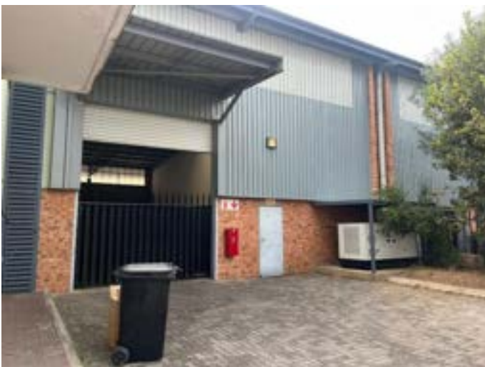
Photo 1: Entrance to Unit 17 of the Linbro Business Park
