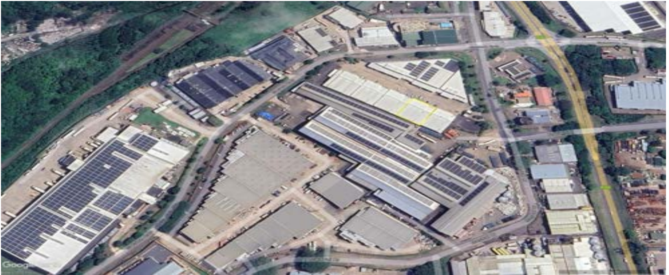
Figure 2: Aerial View of the Mount Edgecombe industrial area and South Group, Durban Facility
