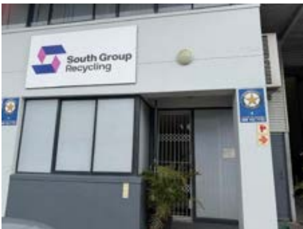
Photo 1: External of office entrance
