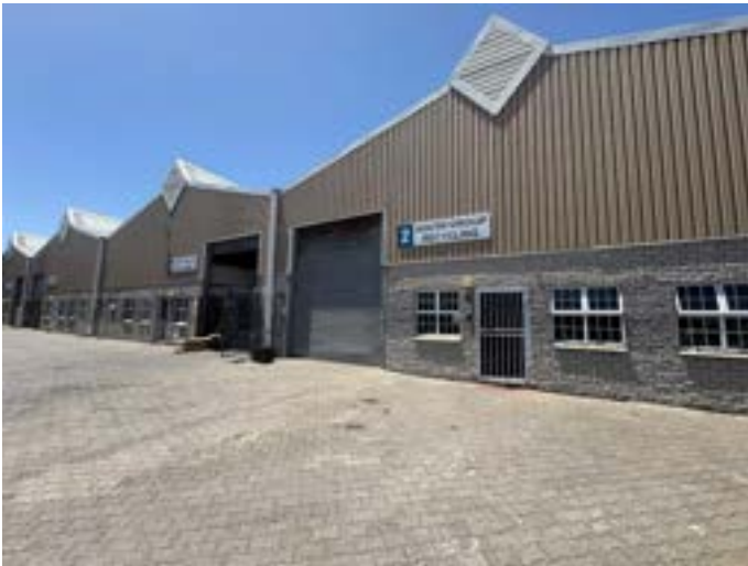
Photo 1: External view of Unit 2 in the Marconi Estate, leased by SGR
