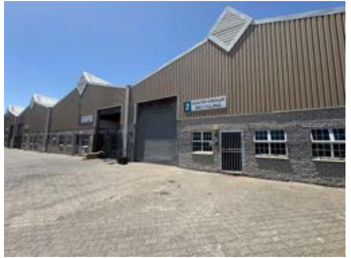
Photo 2: External view of Unit 2 in the Marconi Estate, leased by SGR
