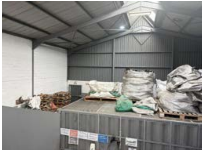
Photo 6: General view of warehouse and operational areas
